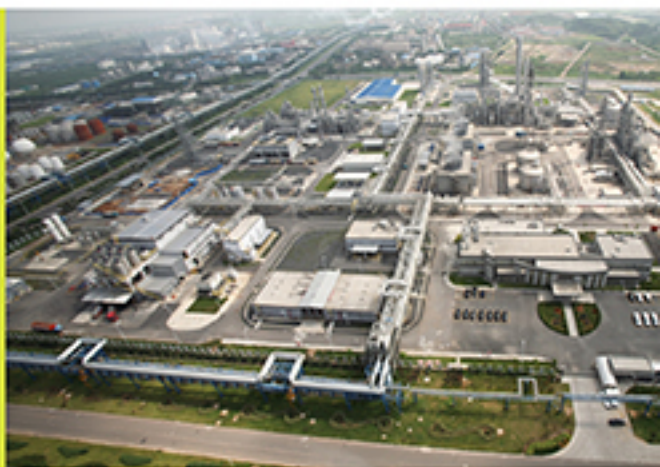
Celanese Nanjing Integrated Chemical Complex.
