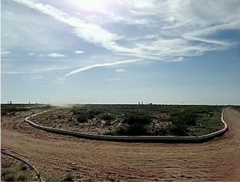
**Lighter With Robust Options** — A 30-foot section of Fiberflex<sup>®</sup>-11 pipe that features Celstran<sup>®</sup> continuous fiber reinforced thermoplastic composites (CFR-TP) weighs only 128 pounds vs. the same length of 12-inch HDPE SDR 9 pipe that weighs 655 pounds. The pipe system offers several robust coupling/connector options, including a two-bolt patent-pending quick coupling design.
